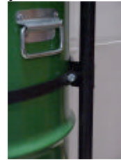
Hoop locked with nut and bolt
